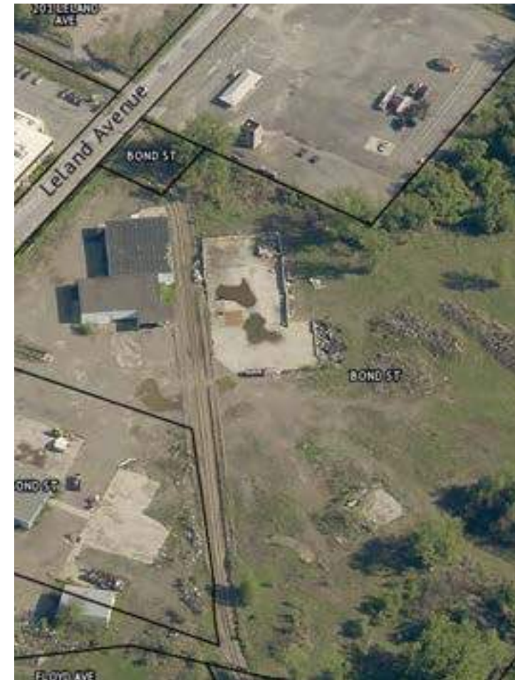
Aerial of Former Utica Alloy Site.
